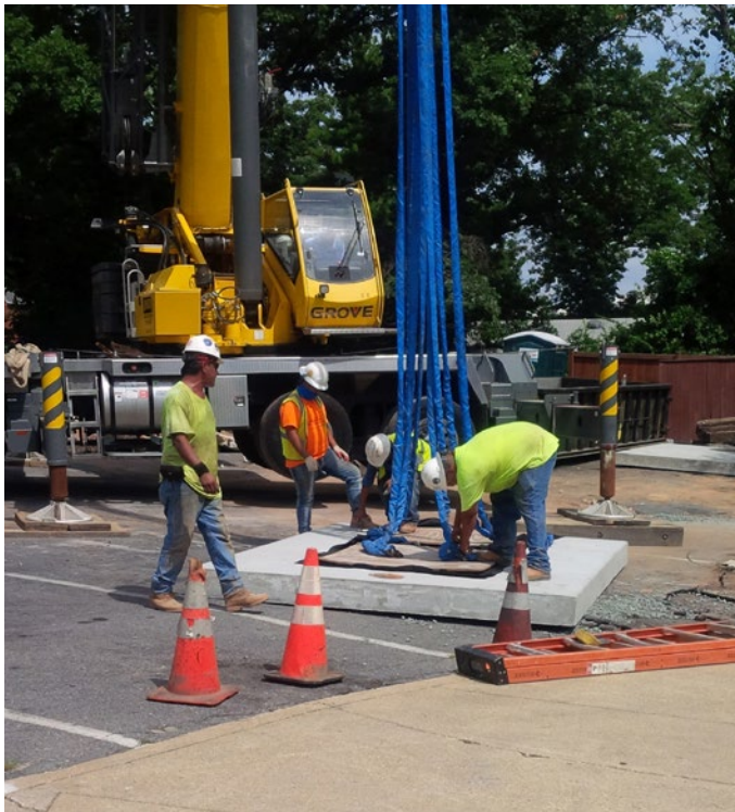
Construction at St. Ambrose Church
