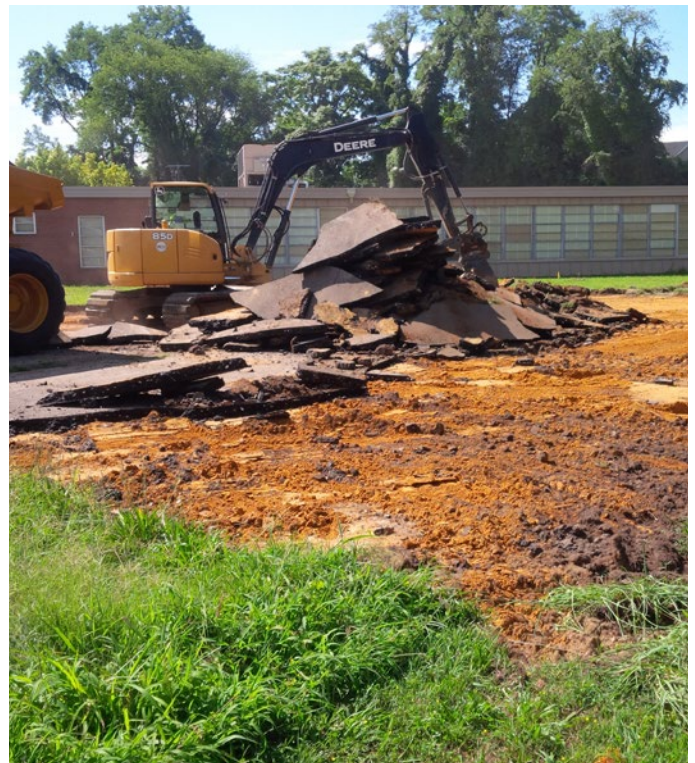
Capitol Heights Elementary School pavement removal
