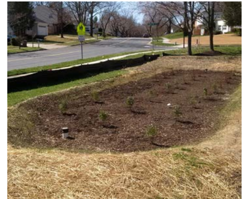
Completed Bioretention facility at Kettering Baptist Church.
