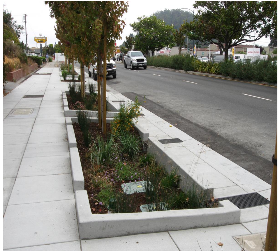
Street retrofit with green filtering devices
