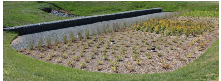
Submerged Gravel Wetland Retrofit Millbrook Pond, Laurel, MD
