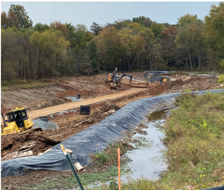
Greenbrook Lake Pond Retrofit, Greenbelt, Maryland
