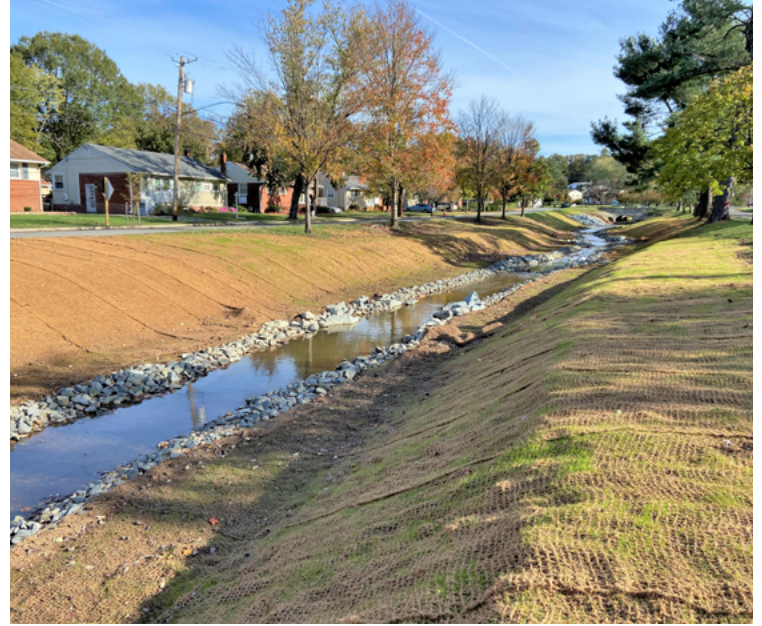
Brier's Mill Run Stream Restoration, New Carrollton, Maryland
