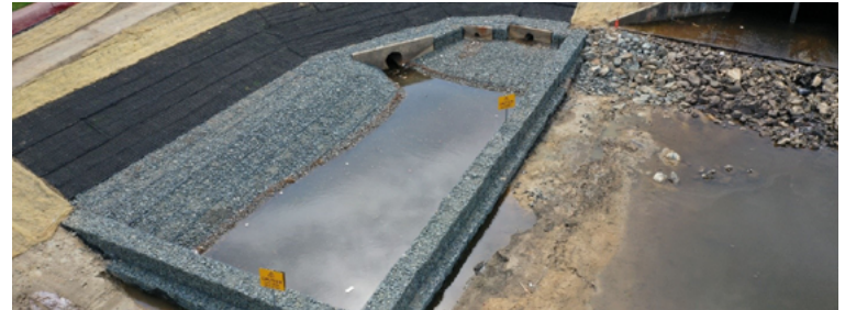
Forebay Construction Lower Laurel Lake at Granville Gude Park
