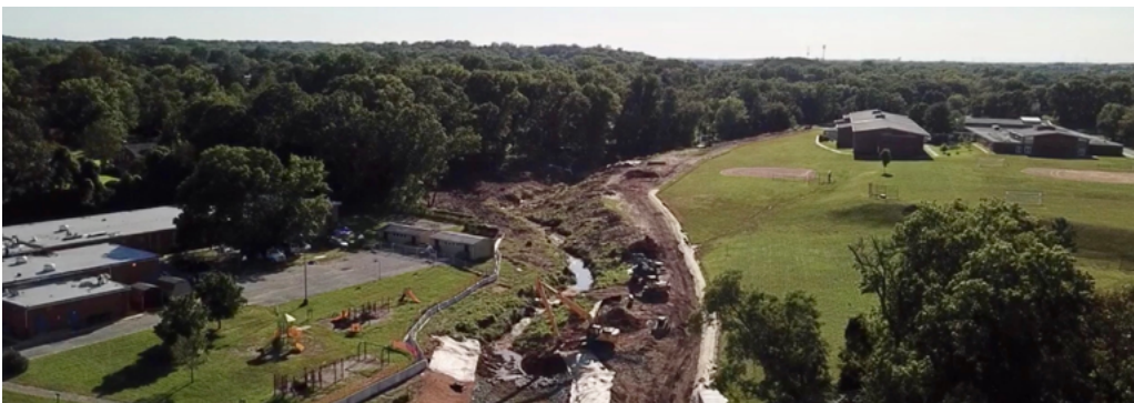
Drone images capture the progress of Oaklands Stream Restoration Project in the City of Laurel.
