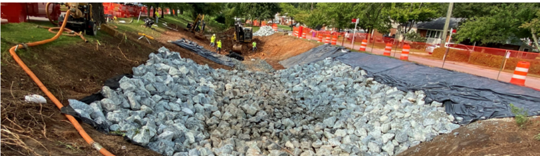
Briers Mill Run Stream Restoration in New Carrollton, Maryland
