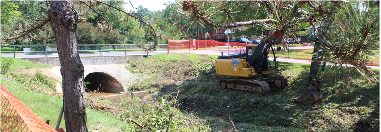
CWP work is underway for stream restoration construction at Briers Mill Run, with plans to install new walking paths in the months following.
