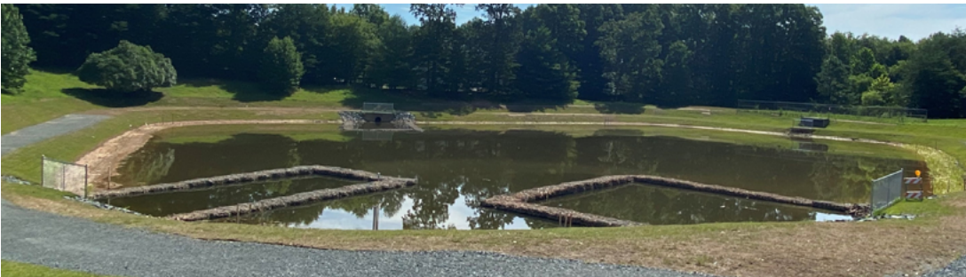
Glenn Estates Pond Retrofit in Lanham, Maryland
