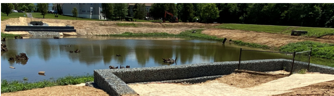
Lakeview Pond Retrofit Gabion Wall Construction in Bowie, Maryland
