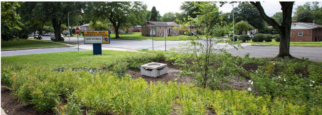
Walker Mill Middle School Micro-bioretenion & Swale
