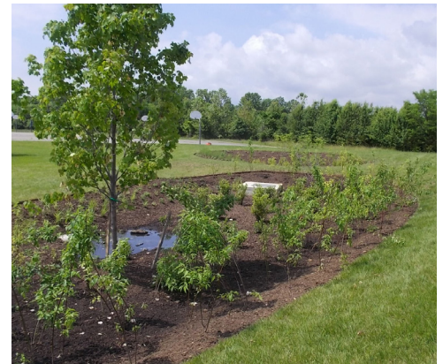
Completed bioretention at the Junior Achievement Finance Park, Prince George's County
