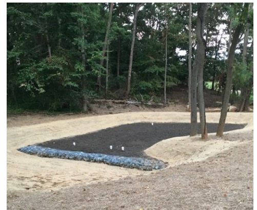
Micro-bioretention at the Cheverly Public Works Yard
