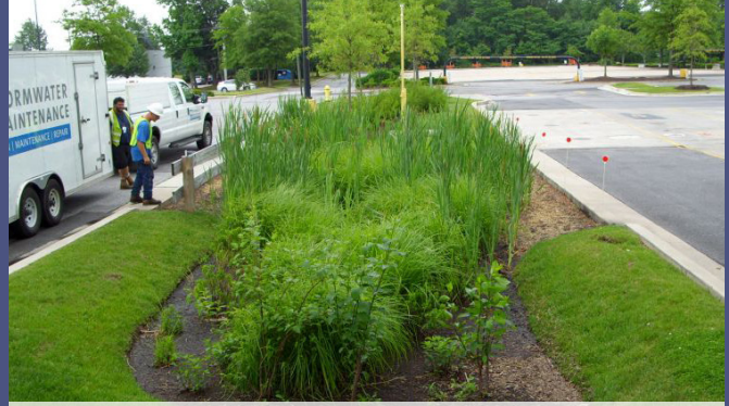
Micro-bioretenion in a parking lot
