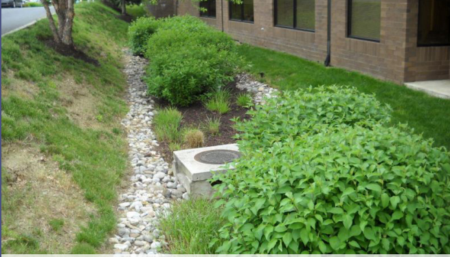
Micro-bioretenion adjacent to a building 3/2011 10/02
