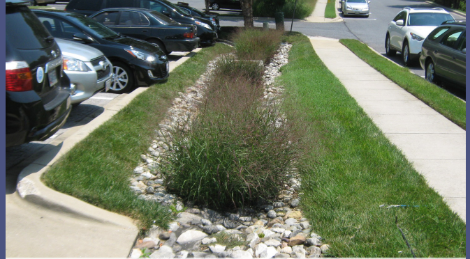
Bioswale adjacent to a parking lot
