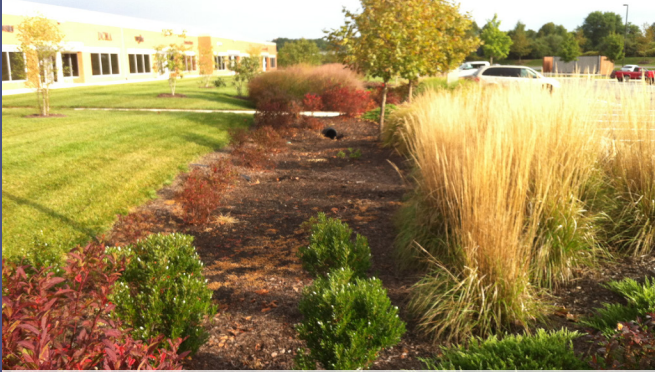
Bioswale in an open space
