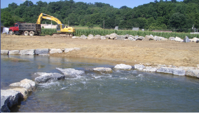
Stream restoration during construction
