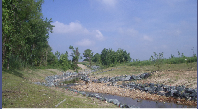
Stream restoration post construction
