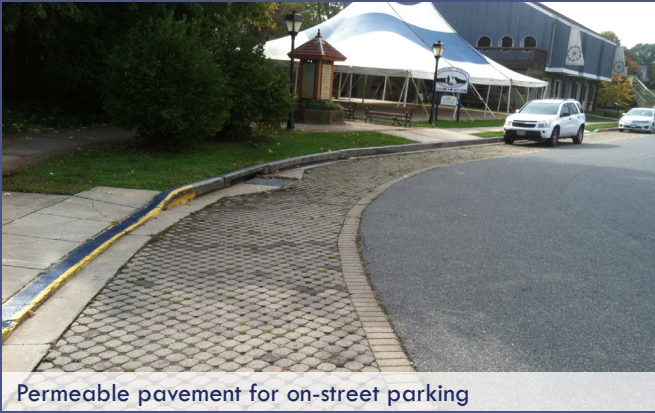
Permeable pavement in a parking lot
